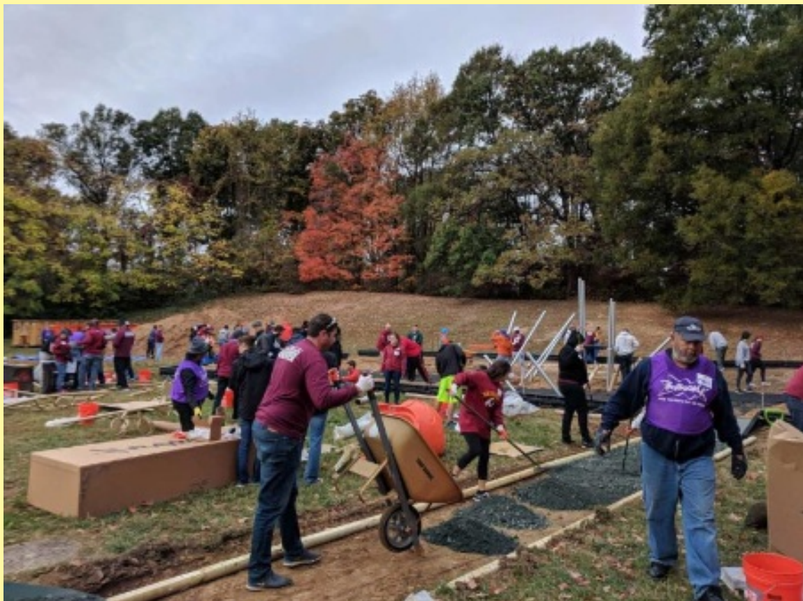
Building a playground for DC Prep
